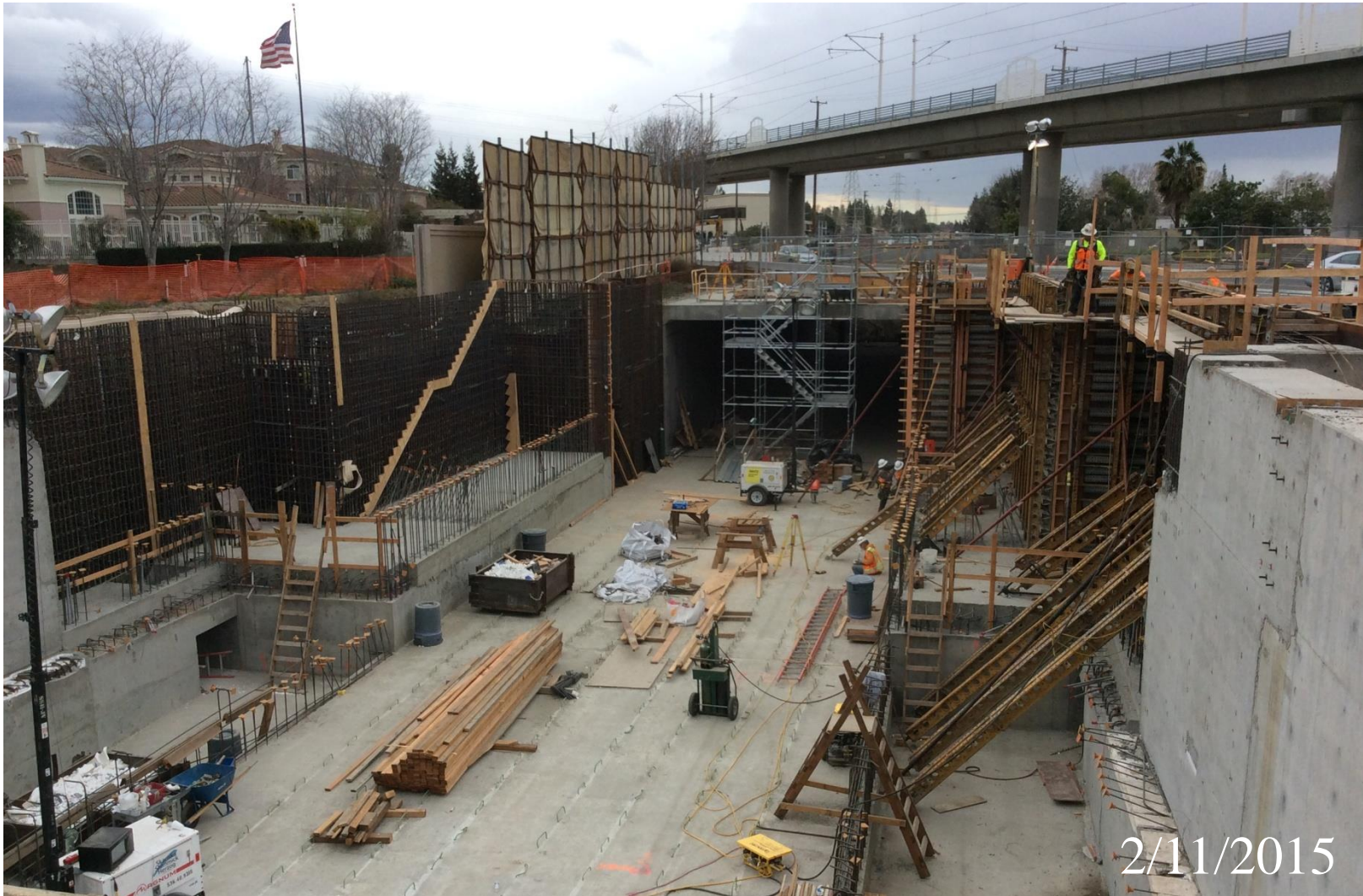
Milpitas station construction
