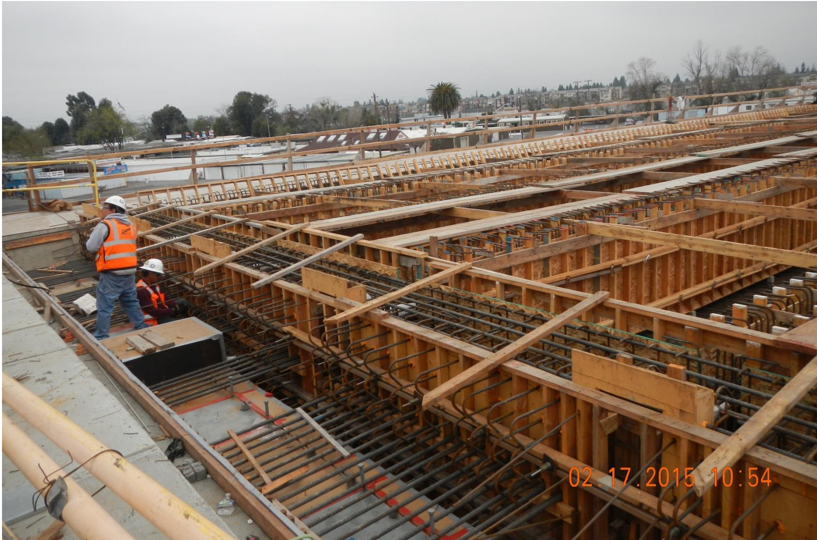
Rebar and formwork for the elevated guideway at the Berryessa Station
