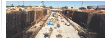
Exterior walls of the station under construction.
