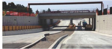
Lowered Warren Avenue with new bridge for the future BART system.
