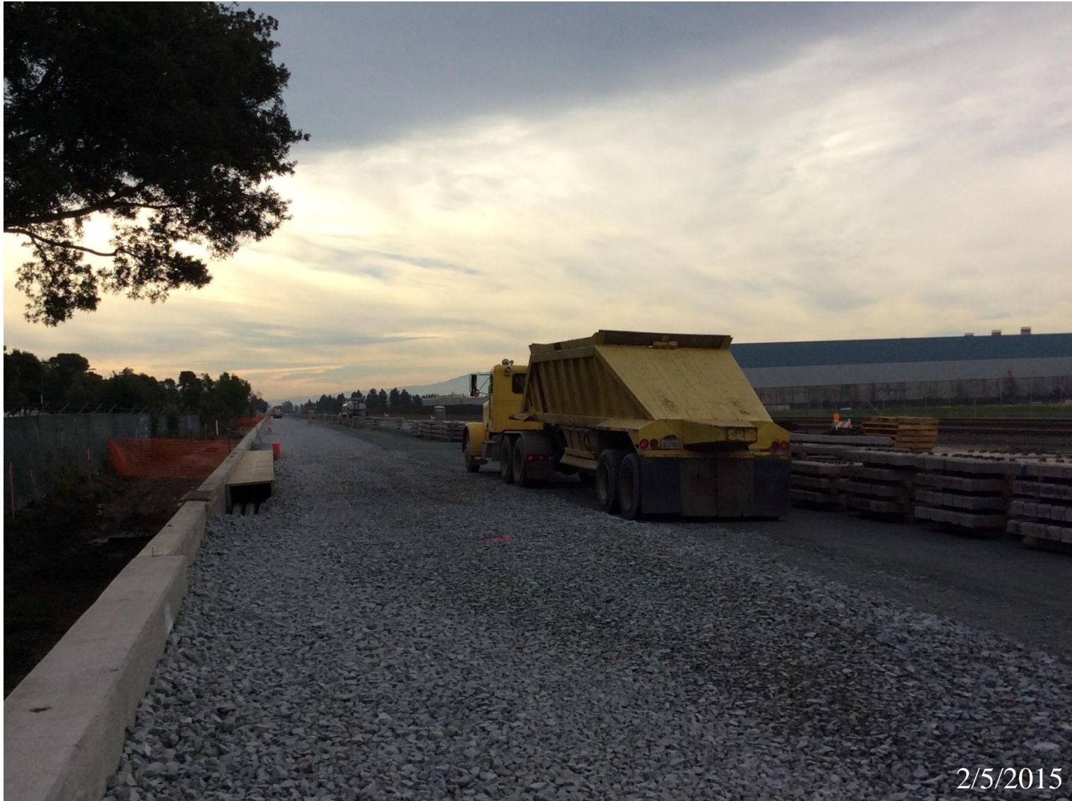
Ballasted guideway and concrete ties in Fremont, looking south
