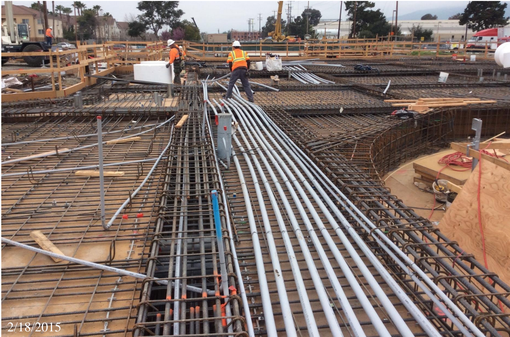
Conduit installation in the concourse deck rebar at the Milpitas Station
