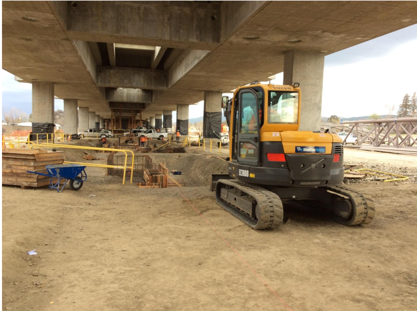
Excavation of elevator pits at the Berryessa Station
