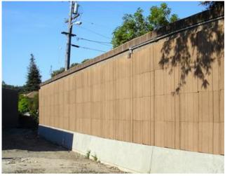
Figure 5-5: Acoustically Absorptive Barrier Tiles
