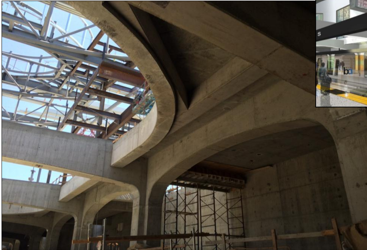
Milpitas Station platform level with concourse level in view above.
